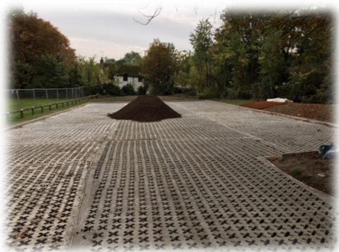
Figure 6 Witchell Car Park extension during construction
