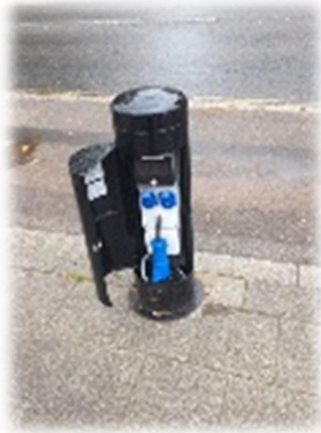
Figure 5 Above ground electrics installed for reliable electrics on the Manor Waste.
