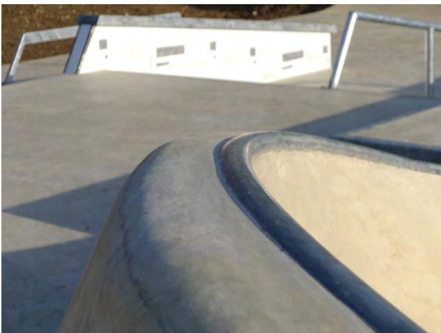
SKATEABLE EDGING IS PROTECTED WITH GALVANISED STEEL EDGING. THIS IS TO AID THE FORM'S USE IN TANDEM WITH CREATING A PROTECTED EDGE.
